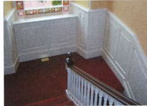
Recently completed staircase with fielded panelling
